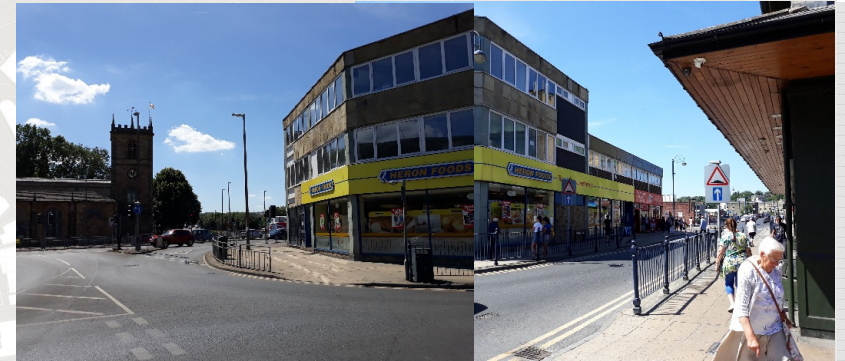
Removal of this dated building could open up the space and aid better links across the town and sustainable travel.
